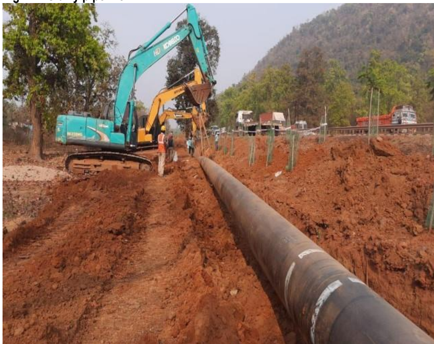
Fig 12 – Slurry pipeline WIP
